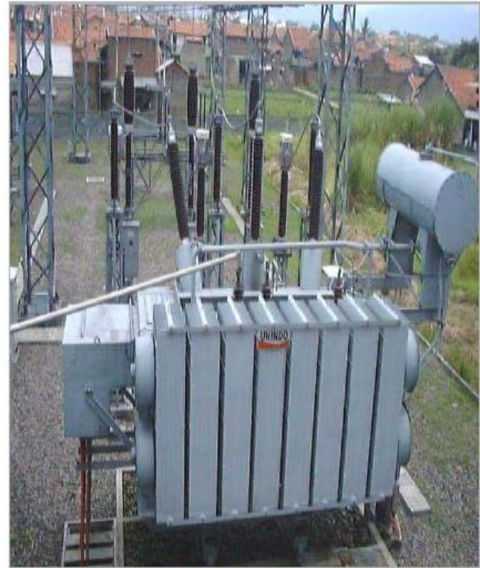
**TRANSFORMATOR TENAGA 150/20 kV 30 MVA**
